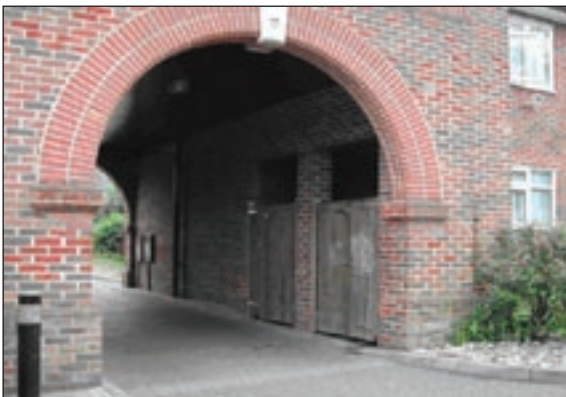
A well-integrated bin store in St Catherine's, Guildford.
