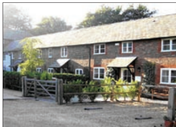
New dwellings in East Horsley with a simple design, sensitive boundary treatment, planting and gravel parking areas, respecting local identity.
