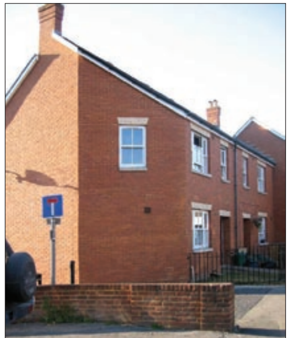
Affordable housing in Stoke Road respects local character.
