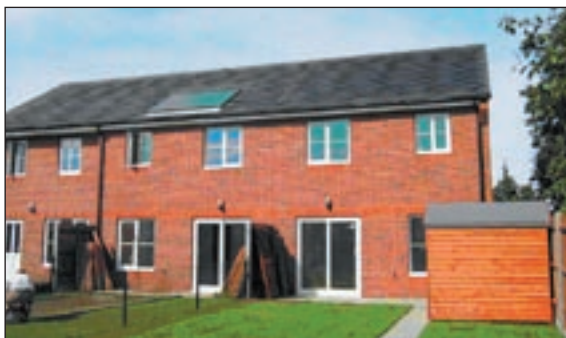
New dwellings at Parsons Green use photovoltaic cells and a solar thermal panel on the roof.
