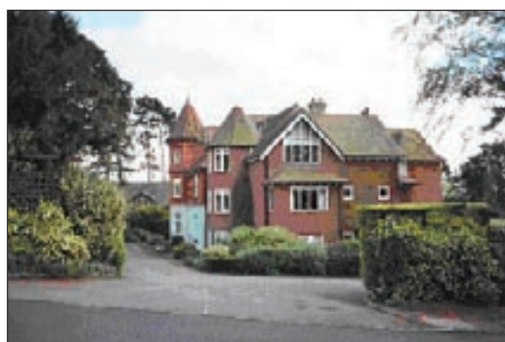
A sensitive extension to an existing historic building in Guildford.
