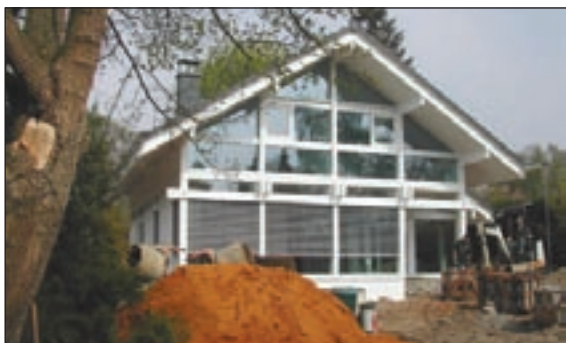
A Huf house under construction.
