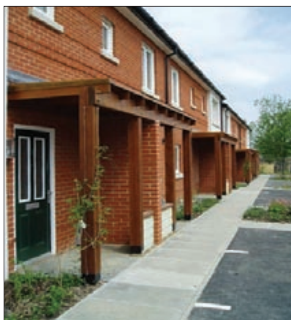
Affordable housing at Queen Elizabeth Park, carefully designed to visually integrate with the overall design of the development.
