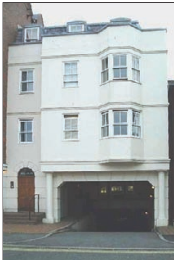
Basement parking integrated within a flatted development.
