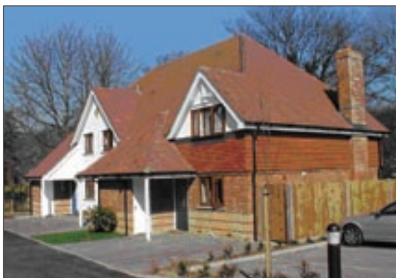
Affordable housing at Barnes Wallis Close, Effingham.
