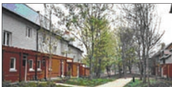
Foot/cycle paths meander through new housing at Queen Elizabeth Park. The permeable surface treatment allows for natural drainage.
