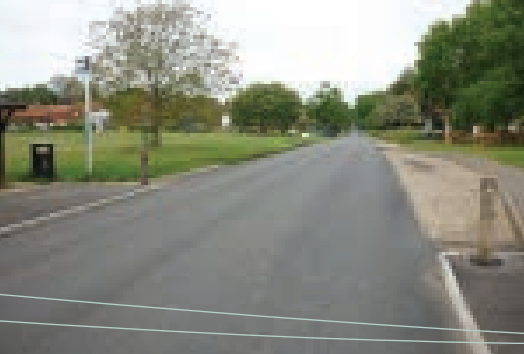
Removing white lines, Shamley Green
