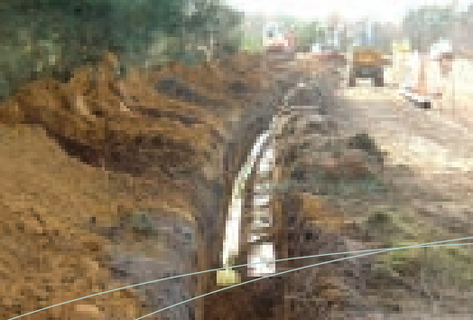
Undergrounding cables, Thursley NNR
