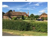
House, now divided. Mid C16 extended to left in late C18 and to right in C20. Timber framed, underbuilt in red brick on rendered plinth, exposed above with red and blue brick infilling. Brick extension to right tile hung on first floor, weatherboarded pentice to left. Plain tiled hipped roof, machine tiled to right over extensions. Two storeys, 3 framed bays with one bay extension to left and over bay extension to right. Ridge stack to right of centre. Mixed casement fenestration,
