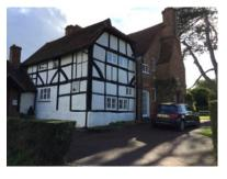
whitewashed infill, plain tiled, half-hipped roof. Red and brown brick to right with some tile hanging and gabled, plain-tiled roof. Old entrance front at right angles to street, new entrance front to rear, parallel ranges with link at right angles between. Rear elevation:- 2 storeys and attics under 2 gabled tile hung casement dormers. Plinth with plat band over ground floor. Regular front of three casement windows on first floor, two windows below under gauged brick
