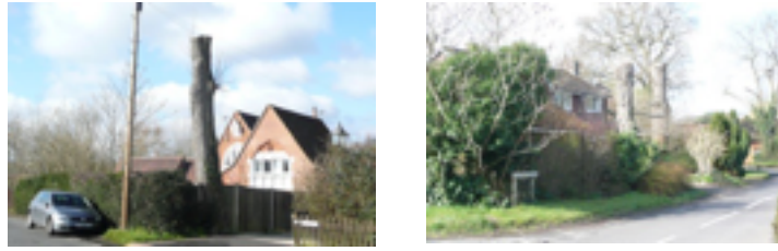
Inappropriate tree pruning
