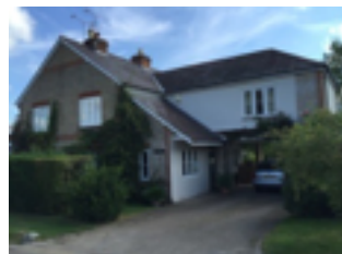
House extension, Silkmore Lane
